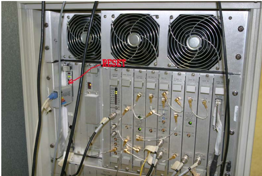
Mercury 300 RESET Button position.
